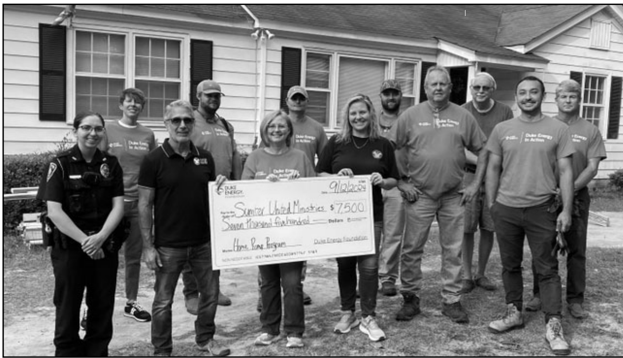
The Duke Energy Foundation is providing $100,000 in grants to 13 organizations in South Carolina to support programs that provide home ramps for low-income senior citizens. Duke Energy Foundation photo
