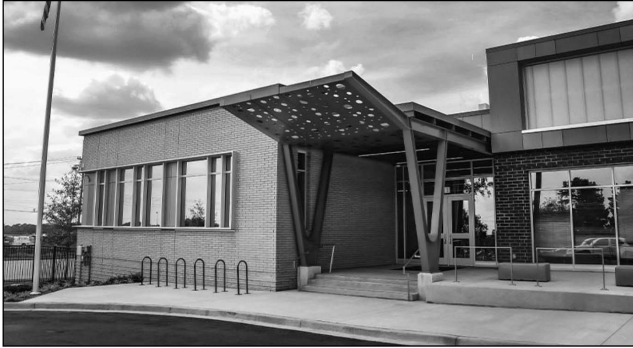
The CTE Innovation Center at Roper Mountain was recently dedicated in late September, exactly one year after groundbreaking for the $12.7 million, 29,145 square-foot facility. Greenville County Schools photo
