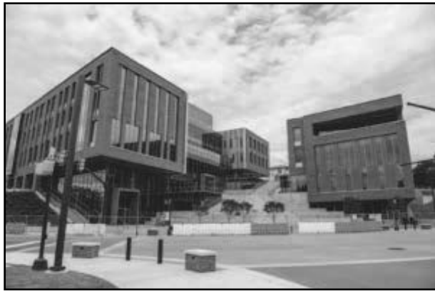
The dual-tower, five-story Wilbur O. and Ann Powers College of Business features 176,000 square feet of building space. As part of the gift, the right structure will be named in honor of their grandson, Chandler L. Burns. Burns was a 2015 graduate of Clemson who died tragically after a short illness in 2016.
