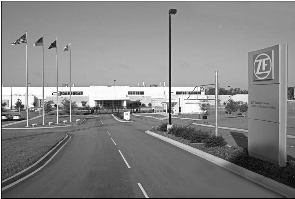
ZF Group recently announced that it will invest $500 million to expand its Gray Court manufacturing facility, creating 400 new jobs. ZF Group photo
