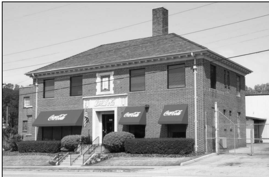
Spartanburg City Council recently approved a development agreement for the redevelopment of the former Coca-Cola distribution center. Coca-Cola Bottling Company photo
