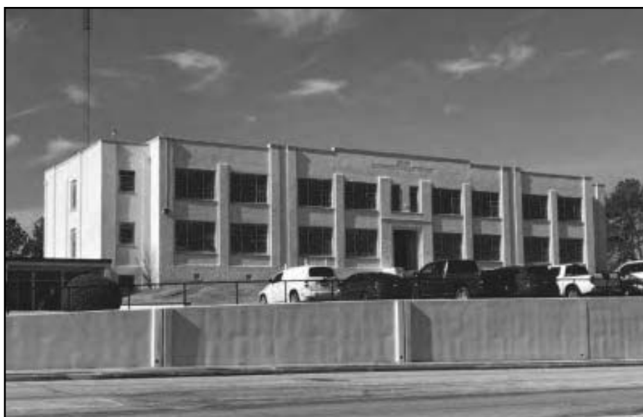
Cumming Street School, among the first school in Spartanburg built for black students, will be added to the City's local Historic Register after a unanimous vote by Spartanburg City Council. City of Spartanburg photo.
