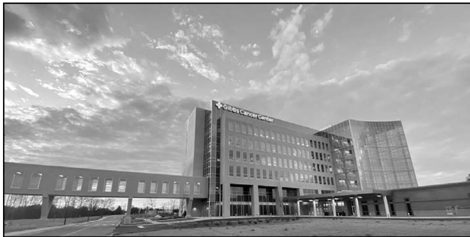
Gibbs Cancer Center at Pelham, a 191,000-square-foot facility in Greer, will begin treating patients later this month.
