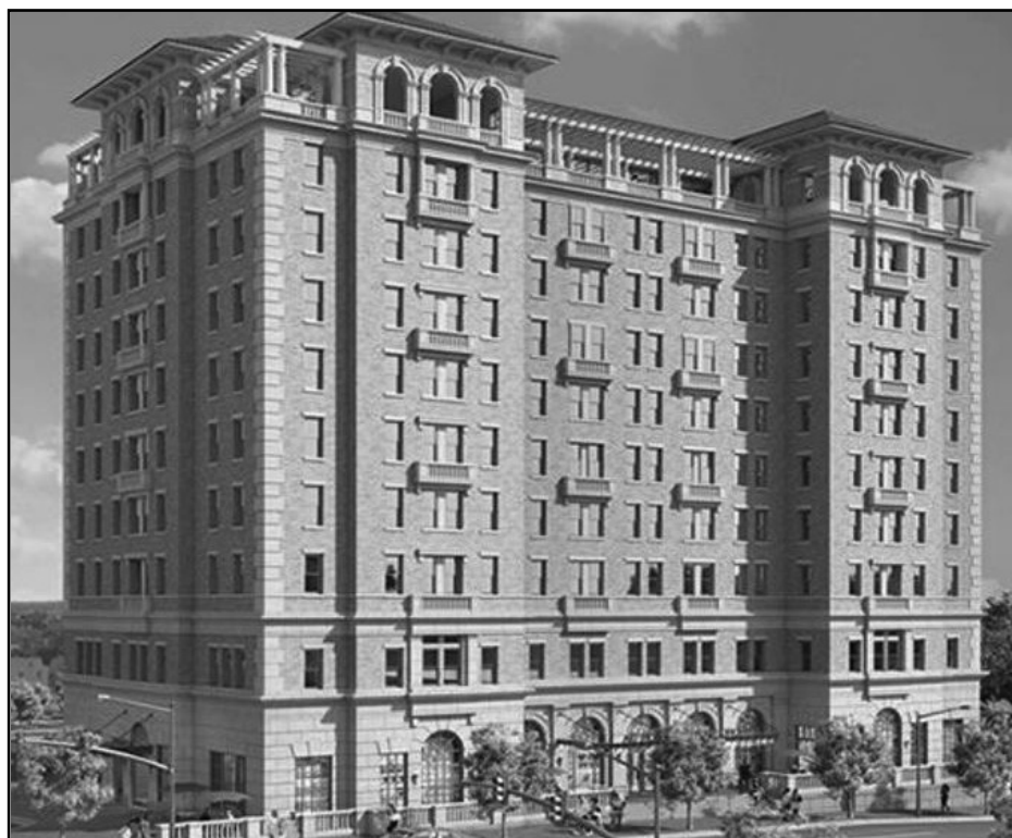
The new AC Hotel Spartanburg will include a rooftop restaurant.
