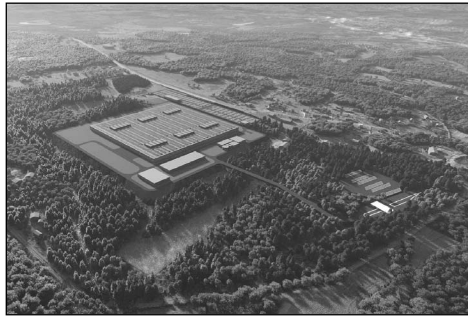
Plant Woodruff will produce batteries for fully electric BMW X Models at Plant Spartanburg. The new Technical Training Center will play a critical role for EV training, and the Woodruff facility will have several sustainability innovations. BMW photo
