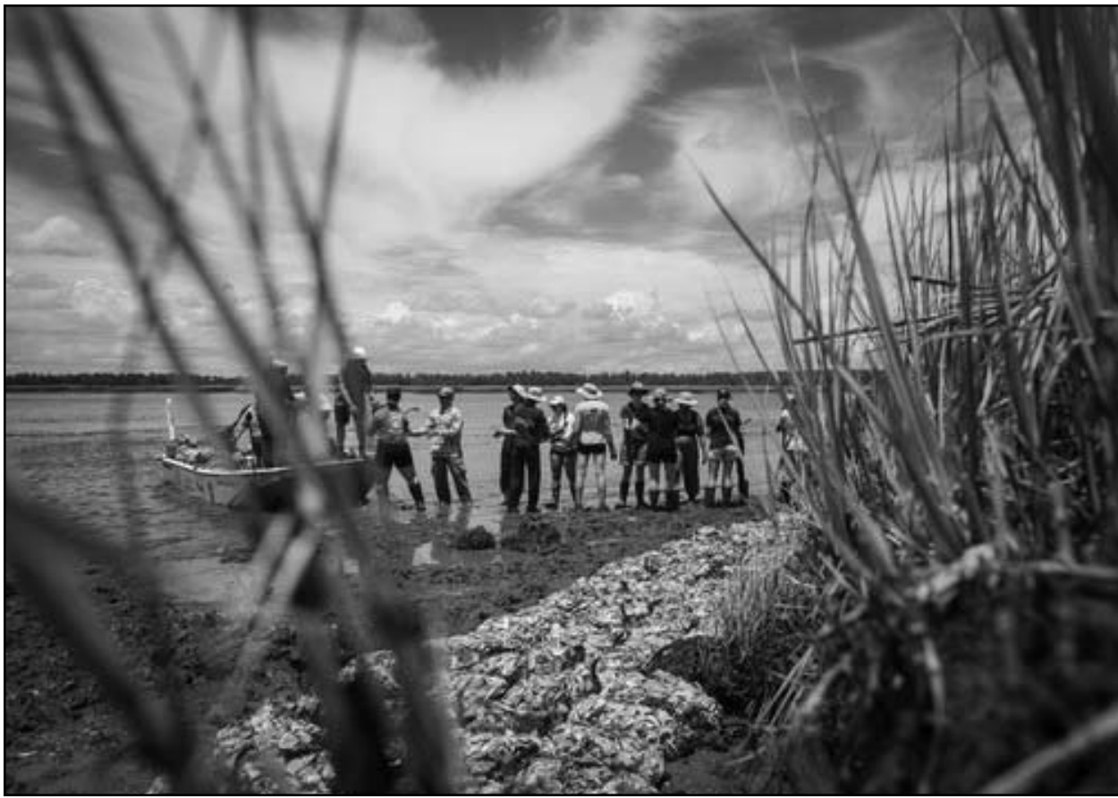
Volunteers form an assembly line to move bags of oyster shells into place along the shoreline. This is one of several strategies that will be employed at Parris Island to improve the natural infrastructure of the area’s shorelines. (Photo: Kaitlyn Hackathorn/SCDNR)
