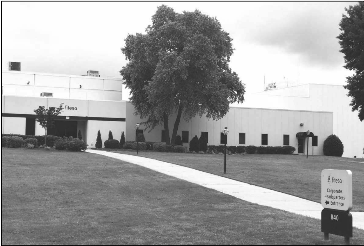
Fitesa is expanding its Simpsonville plant, investing $100 million and creating 40 new jobs.
